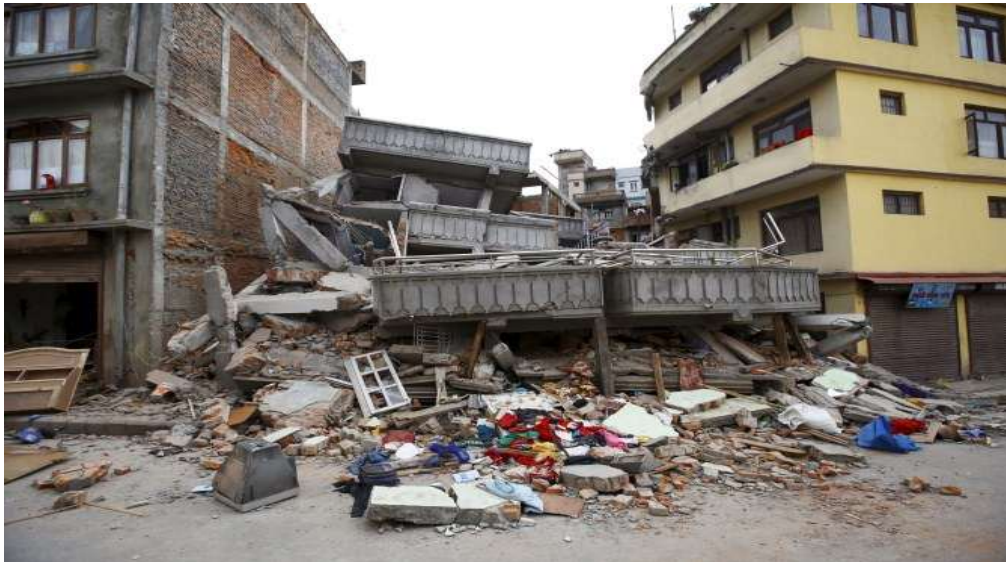
Fig. 6: Complete collapse of a residential building due to Nepal 2015 Earthquake
