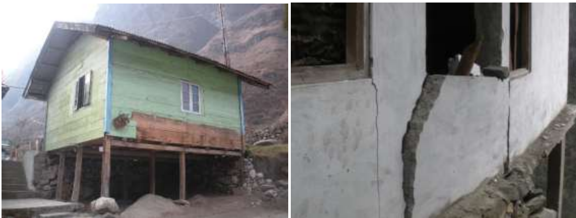
Fig. 7: Buildings status soon after Sikkim 2011 earthquake; (a) Constructed in traditional techniques and locally available material and (b) Constructed by modern material without engineering considerations
